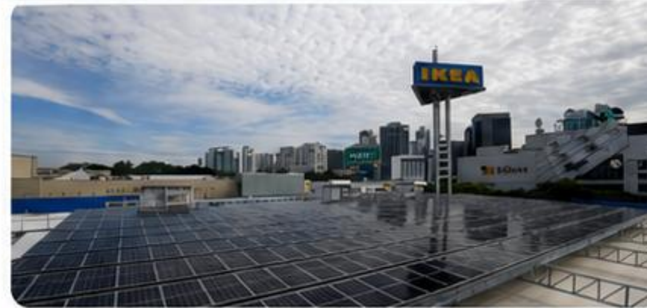
Solar Rooftop Installation
